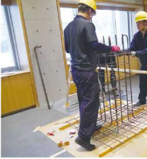
柱鉄筋組立て
