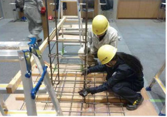
柱鉄筋組立て
