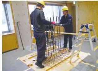
柱鉄筋組立て
