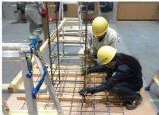
柱鉄筋組立て
