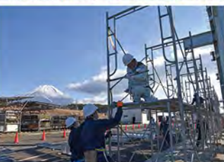
仮設足場組立て
